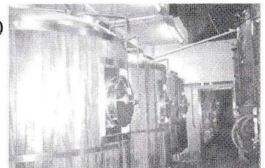
Inside the renovated Brewery
