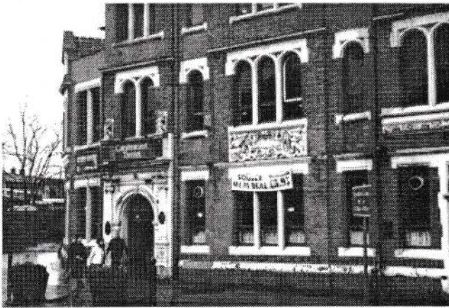
One of the most prominent pubs in Stockport - the Chestergate Tavern in its current dilapidated state
